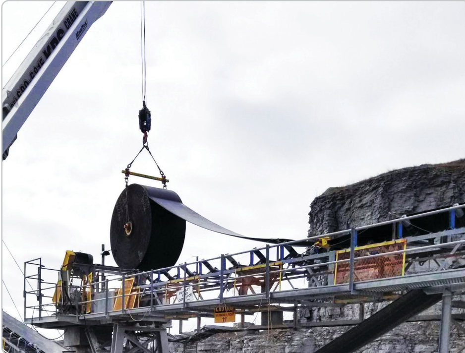
Only properly rated crane should be used.
